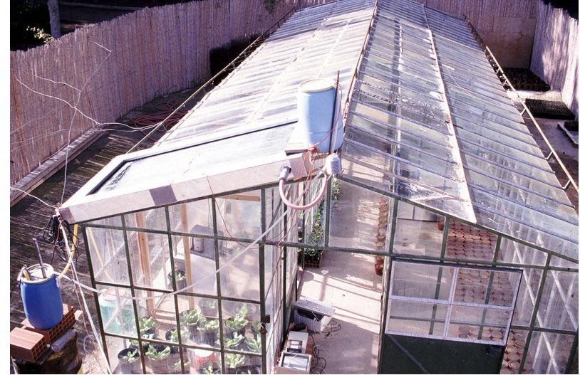
Greenhouse system with integrated water desalination
