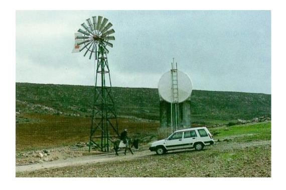
**Mechanical Wind Energy for Water Pumping**
