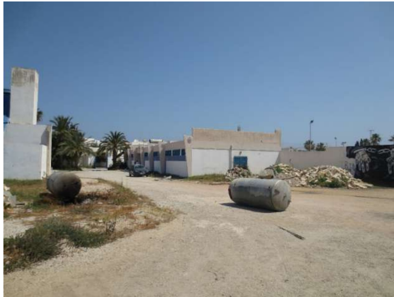
Figure 7: The building next to the swimming pool
