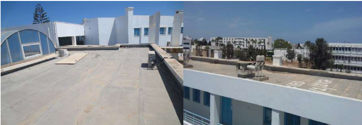
Figure 22: Rooftops for Higher Institute of Biotechnology De Monastir
