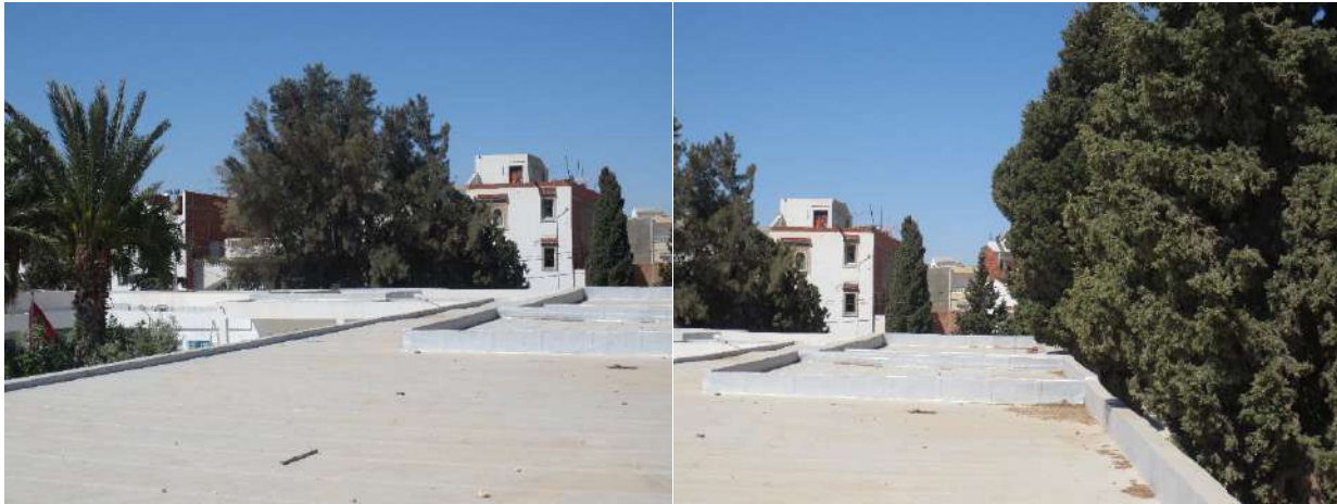
Figure 10: The school rooftops are shaded by surrounding trees
