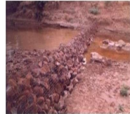
Gabion structure in a stream bed
